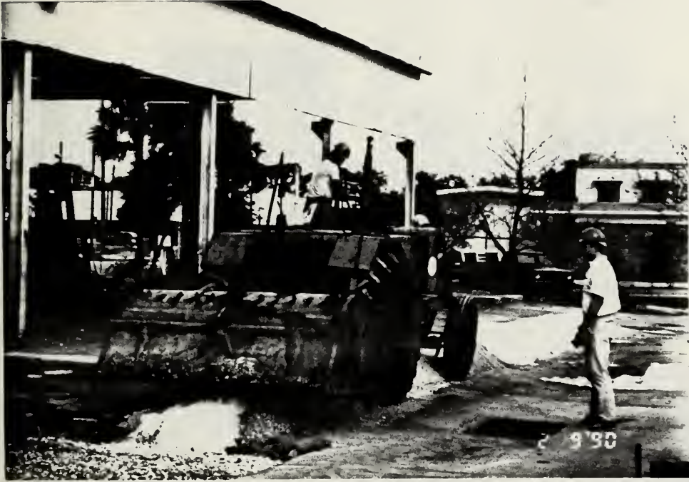
Figure 2.10 Soil Stabilizer Placement
